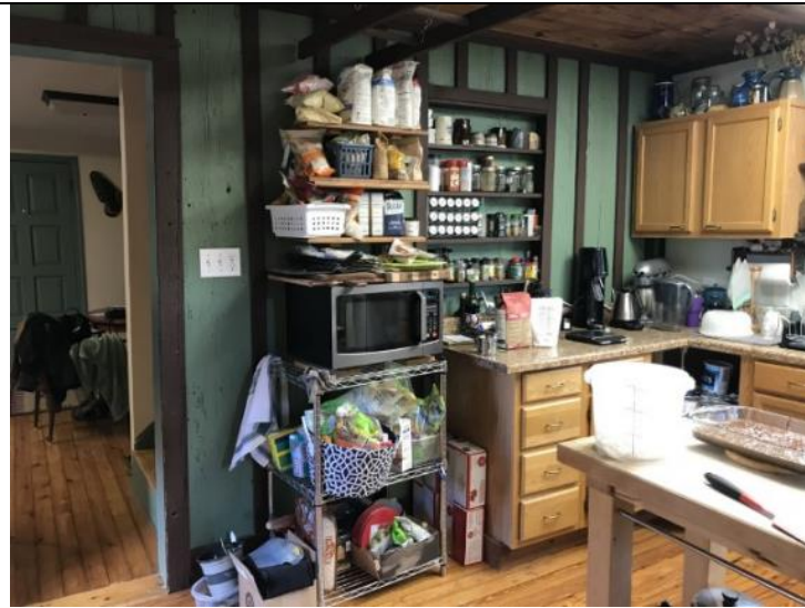
WV_Jefferson_County_Susan Thornton House_0010 Susan Thornton house kitchen addition to original board-and-batten siding. View to northeast.
