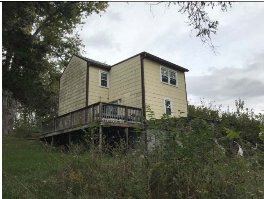
WV_Jefferson_County_Susan Thornton House_0004 Susan Thornton house view southeast to northwest.
