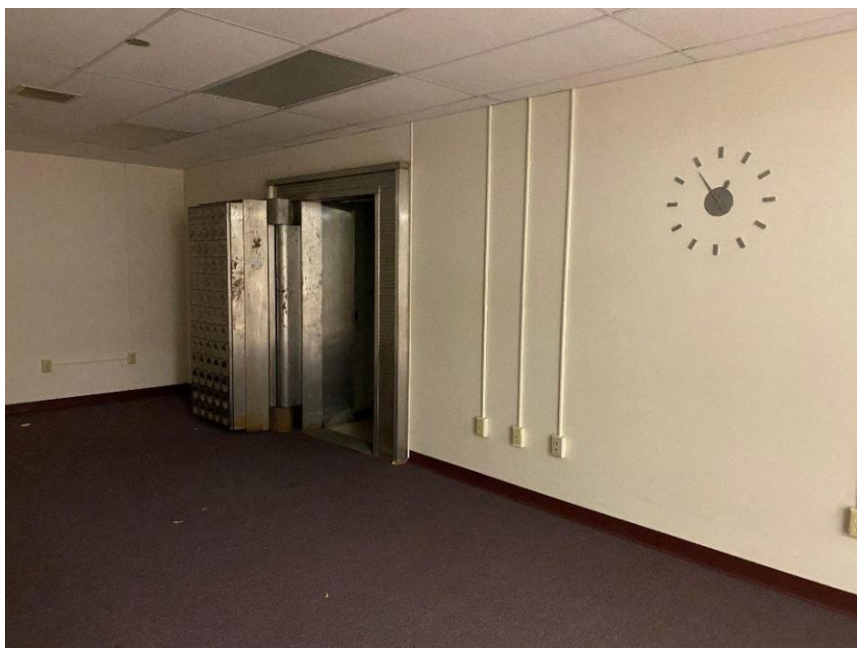
Photo 28: Interior, basement (first floor) vault, camera facing northwest
