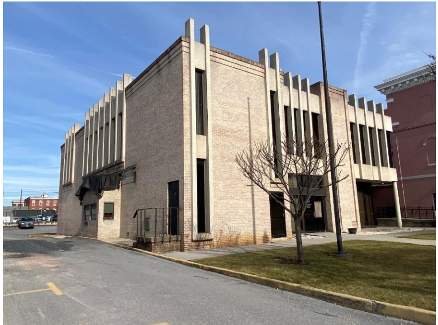
Photo 2: Southwest oblique, camera facing northeast.
