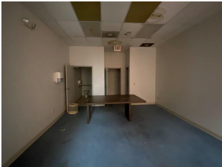
Photo 21: Interior, second floor jury room, camera facing west.
