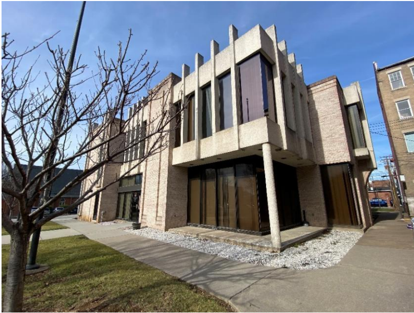
Photo 7: Northeast oblique, camera facing southeast.
