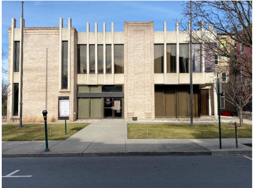
Photo 1: South Façade (right), camera facing north.
