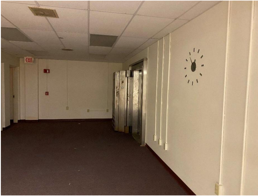
Photo 29: Interior, basement (first floor), camera facing west.
