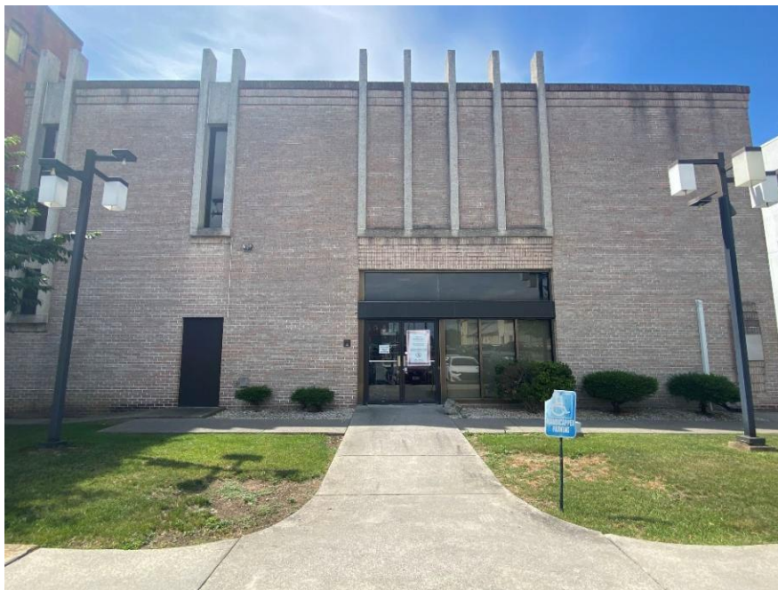
Photo 4: Rear (north) elevation, camera facing south.
