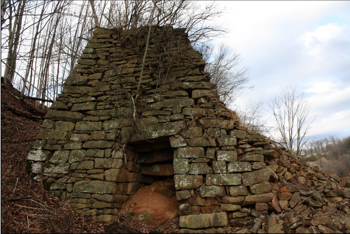
Photo 1. Southwest elevation of the Valley Furnace, facing northeast.
