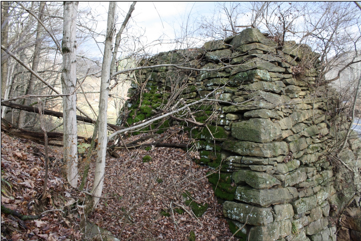
Photo 4. North and west elevations, facing east.
