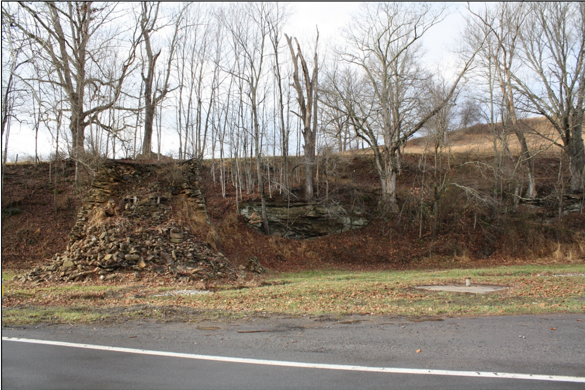
Photo 7. South elevation of furnace, facing north. Note the concrete picnic pavilion pads.
