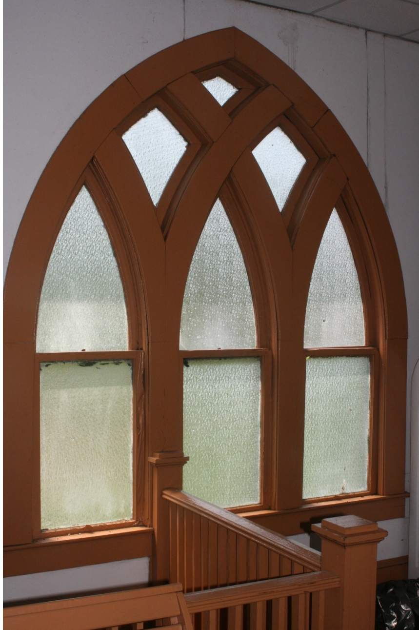
Photo 7 of 10: Detail of sanctuary showing oversized lancet-arched window centered on the south elevation, looking south
