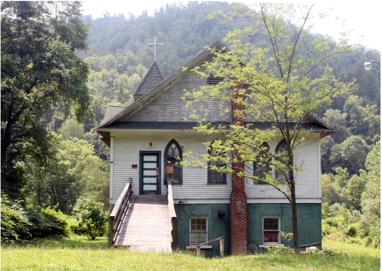
Photo 2 of 10: Rear elevation, looking south, showing massing, including non-historic handicapped ramp
