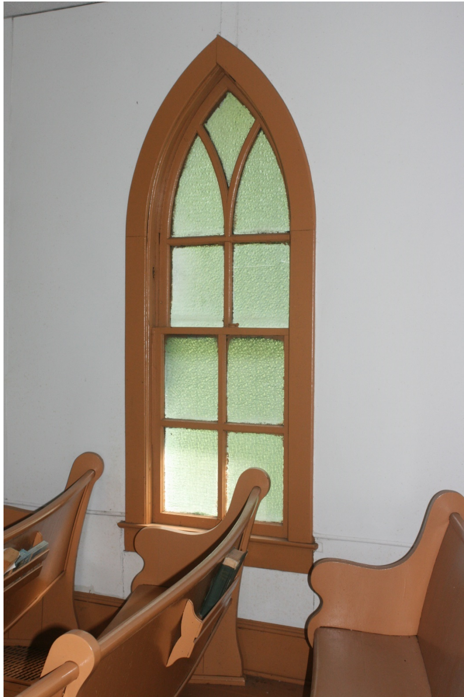
Photo 6 of 10: Typical lancet-arched side window, looking east and showing "snowflake" glazing and typical trim, looking east.
