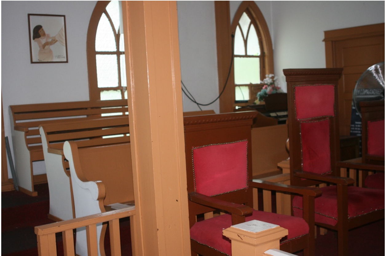
Photo 4 of 10: View of sanctuary, looking northeast and showing support posts, fenestration, pews, etc.
