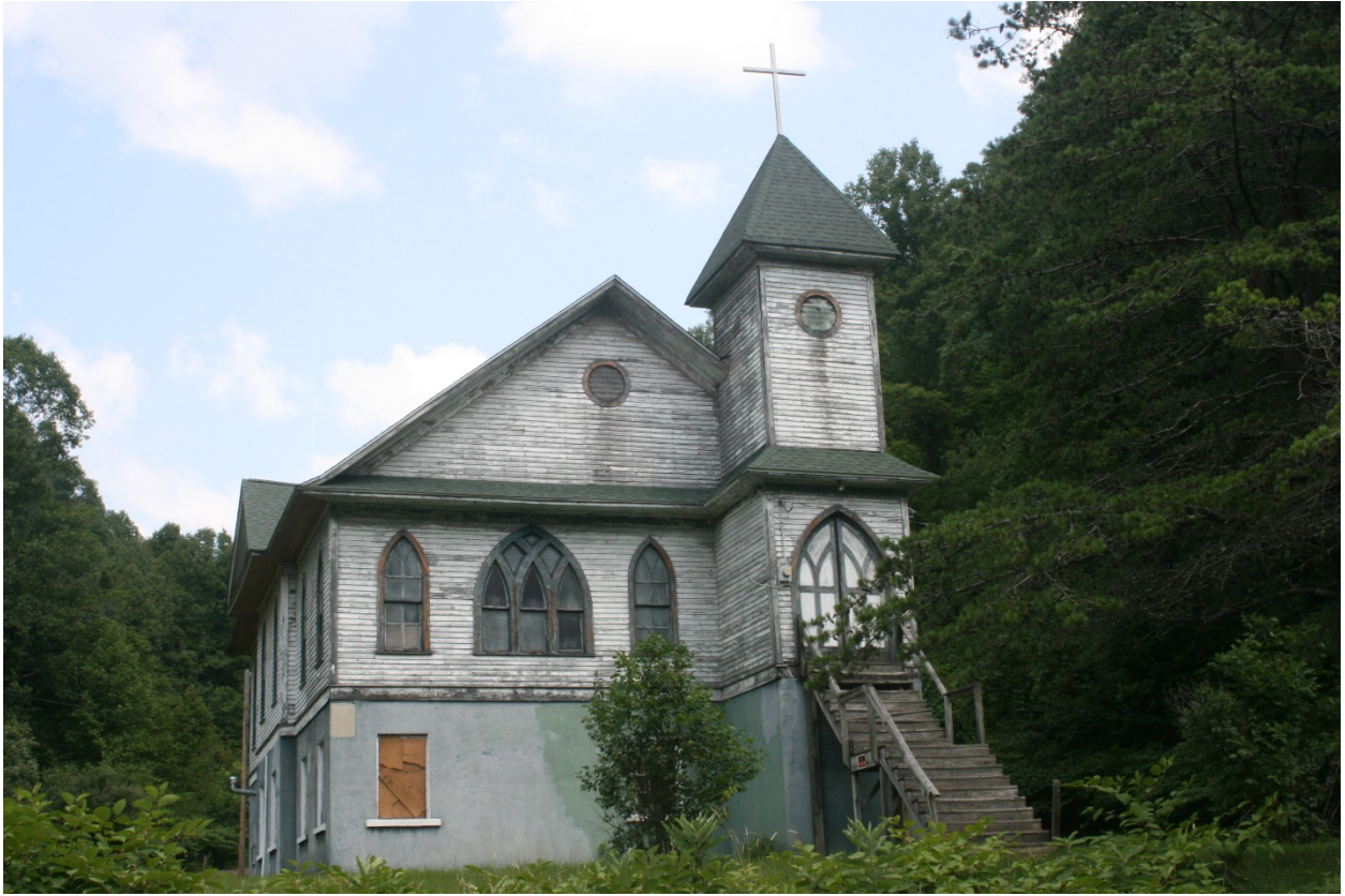
Photo 1 of 10: Façade, looking north
