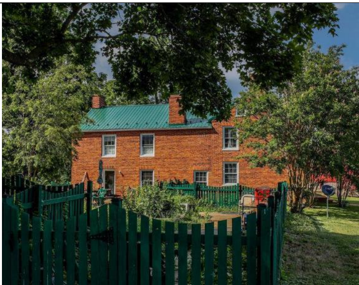
Photo 5. WV_Jefferson_County_James Osbourn Farm_0005
