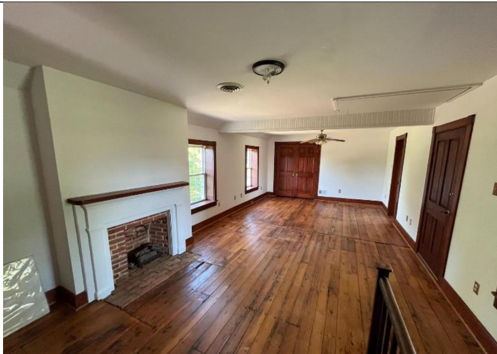
Photo 16. WV_Jefferson_County_James Osbourn Farm_0016 James Osbourn house, second floor addition looking west.
