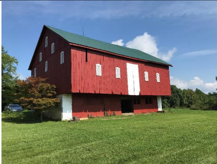
Photo 7. WV_Jefferson_County_James Osbourn Farm_0007
