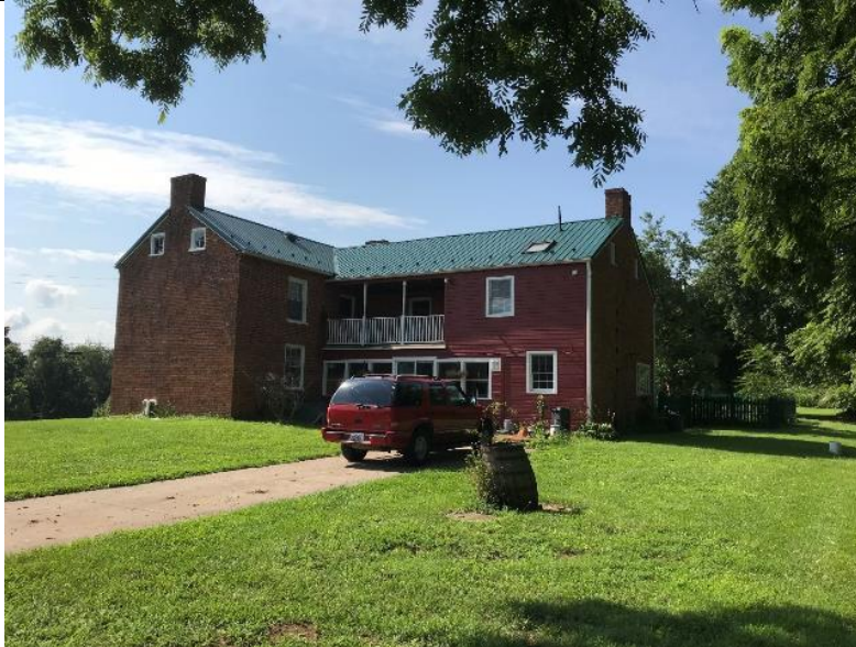
Photo 3. WV_Jefferson_County_James Osbourn Farm_0003
