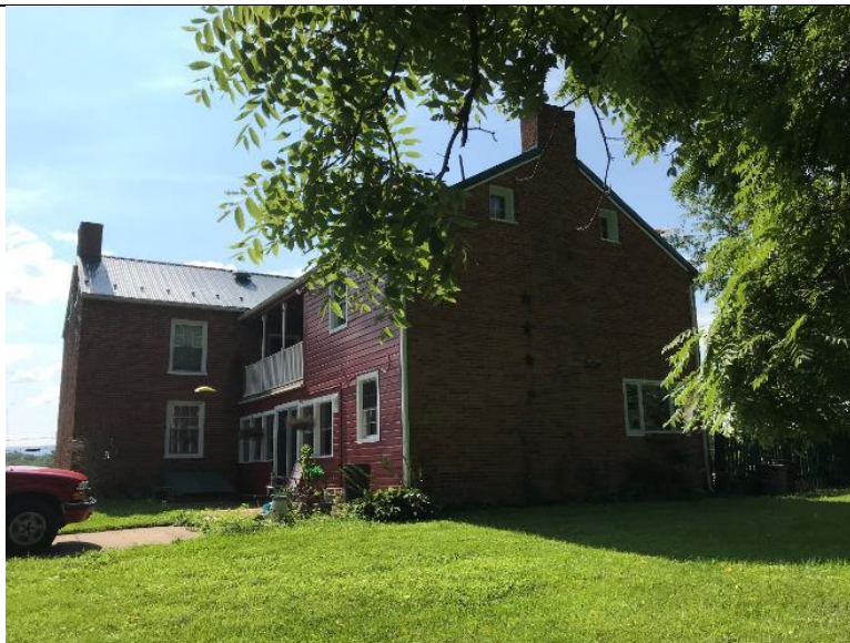
Photo 4. WV_Jefferson_County_James Osbourn Farm_0004.
