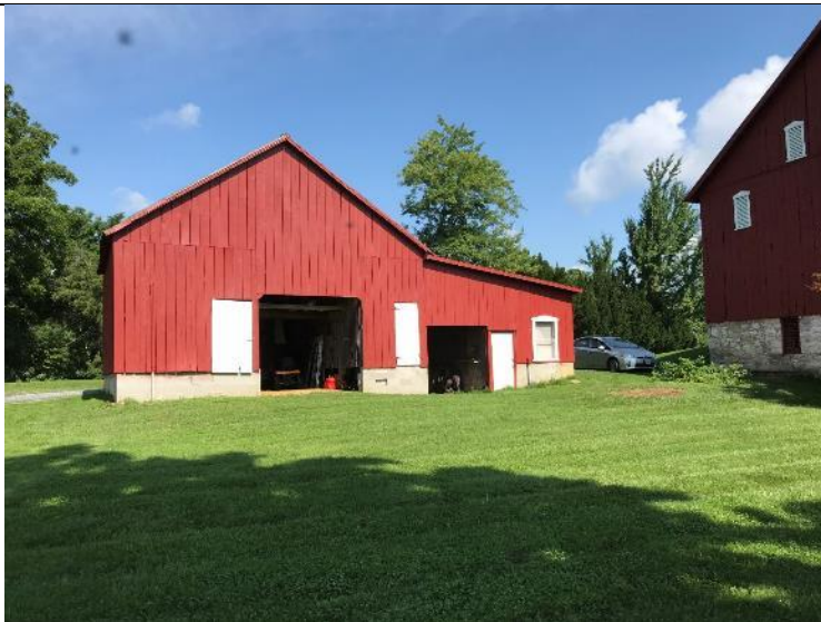
Photo 6. WV_Jefferson_County_James Osbourn Farm_0006
