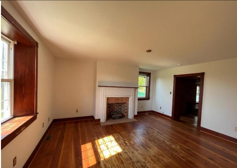
Photo 11. WV_Jefferson_County_James Osbourn Farm_0011 James Osbourn house first-floor front room, south.
