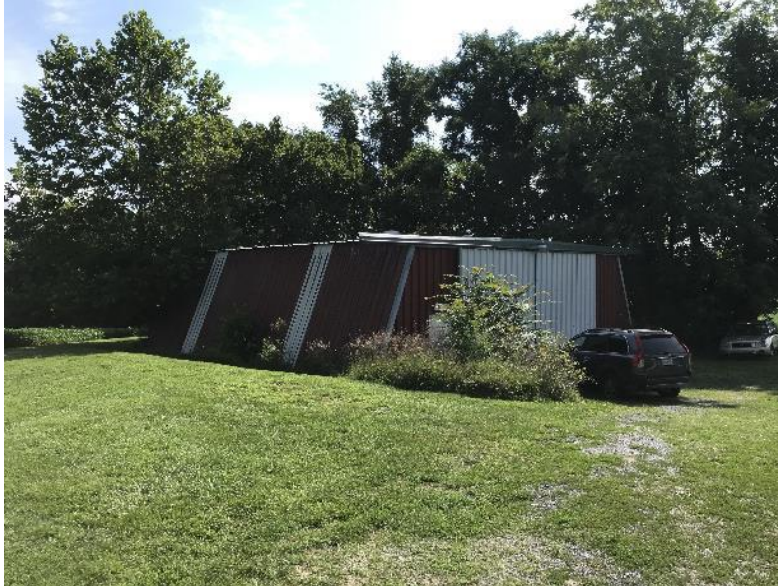
Photo 9. WV_Jefferson_County_James Osbourn Farm_0009
