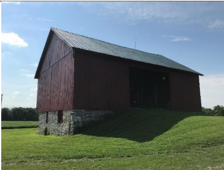
Photo 8. WV_Jefferson_County_James Osbourn Farm_0008
