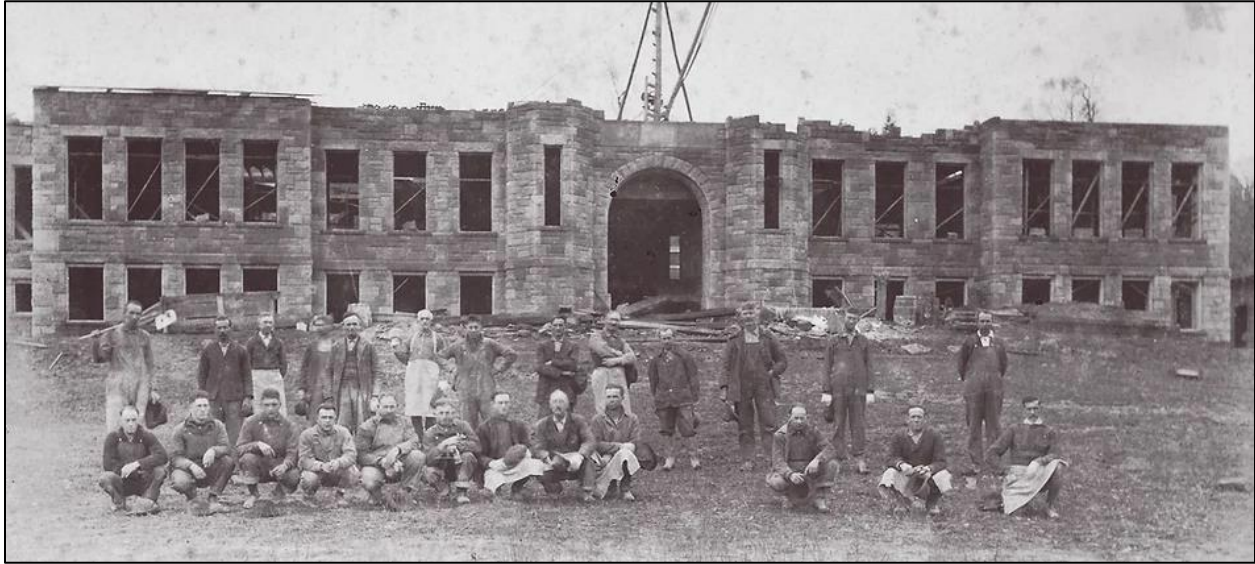
Figure 7. 1921 Image of Calhoun County High School under construction.
