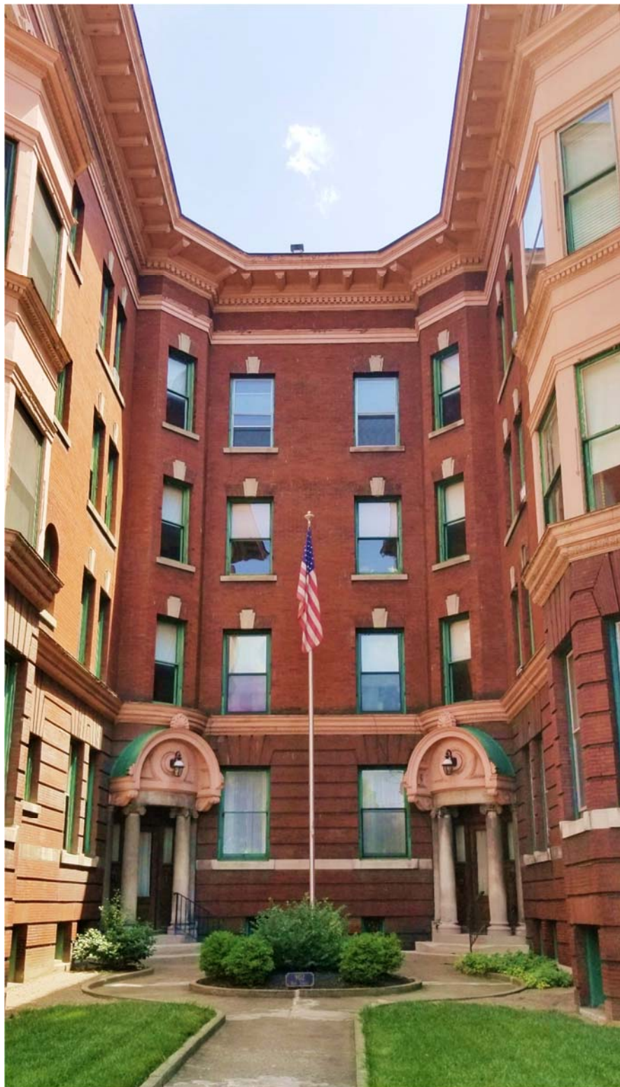
Photo 6: WV_Ohio County_Virginia Apartments_06 View of Virginia Apartments Courtyard
