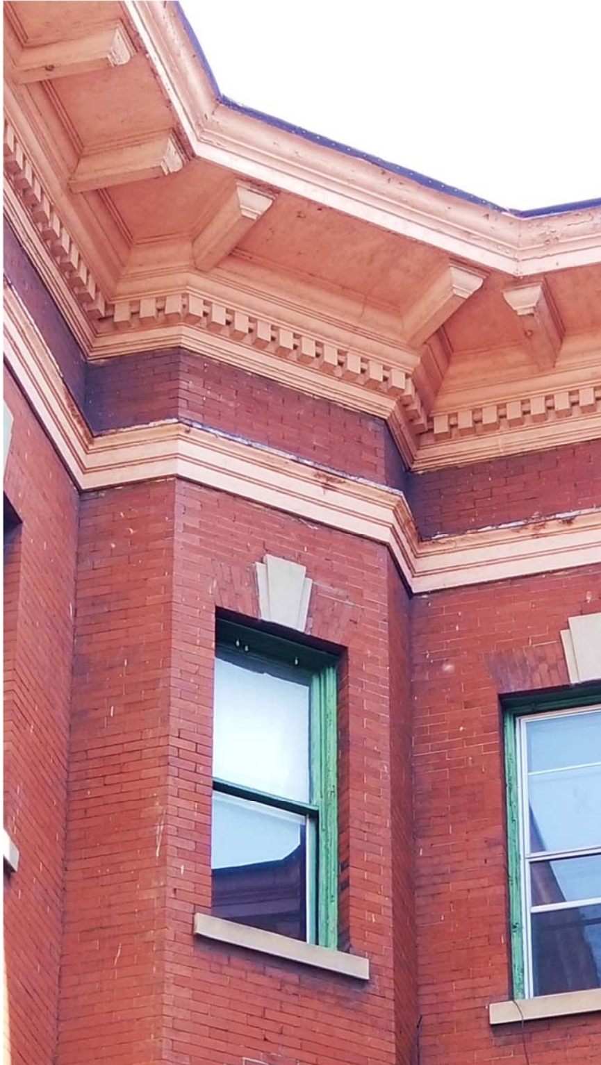
Photo 5: WV_Ohio County_Virginia Apartments_05 Cornice from Courtyard below
