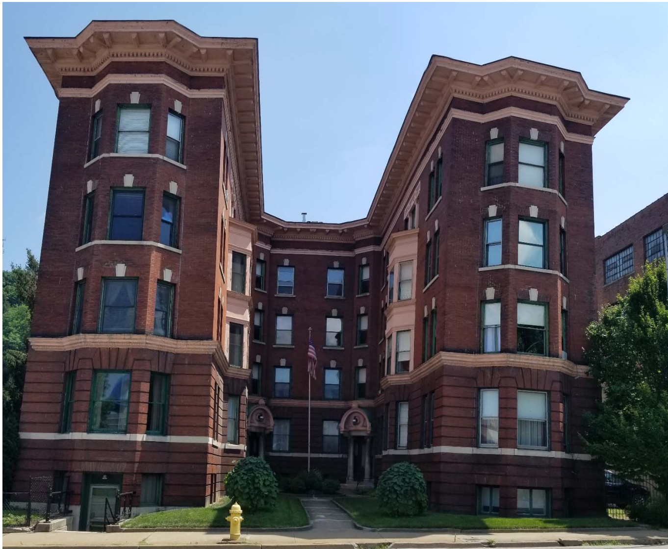
Photo 3: WV_Ohio County_Virginia Apartments_03 View of Virginia Apartments from Main Street
