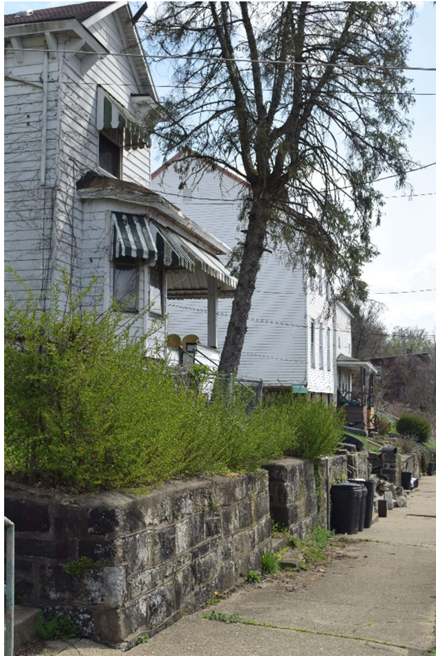
Photo 40. Example of typical sandstone block retaining wall, east Side of Market Street south of Pike Street, looking southeast.
