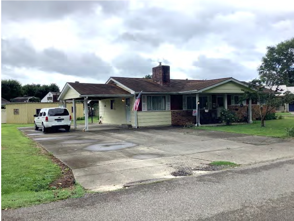
Photograph 25. PU-0007-0109 at 314 Ivywood Street, facing Southwest.
