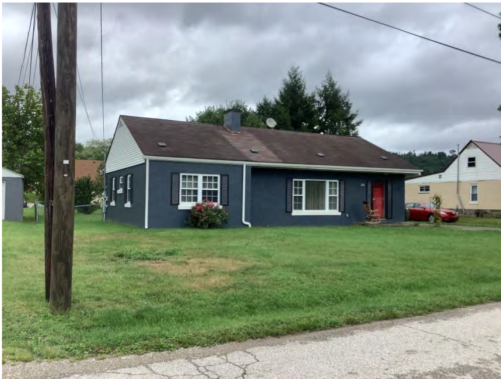
Photograph 26. PU-0007-0105 at 210 Chestnut Street, facing Northeast.
