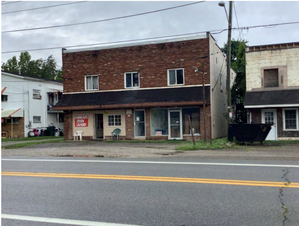
Photograph 15. PU-0007-0148 at 833 Roosevelt Boulevard, facing South.
