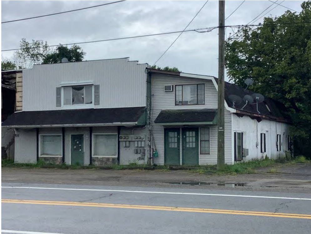
Photograph 17. PU-0007-0149 at 935 Roosevelt Boulevard, facing South.
