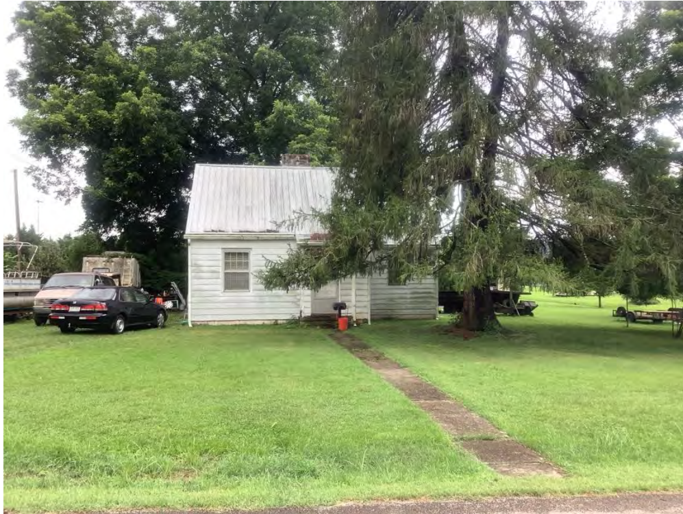
Photograph 19. PU-0003-0365 at 302 Ivywood Street, facing Southeast.
