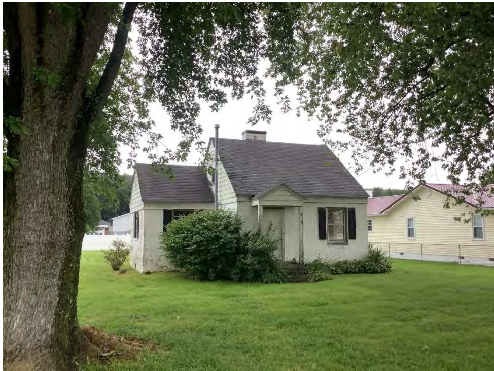
Photograph 23. PU-0003-0417 at 942 Roosevelt Boulevard, facing North.
