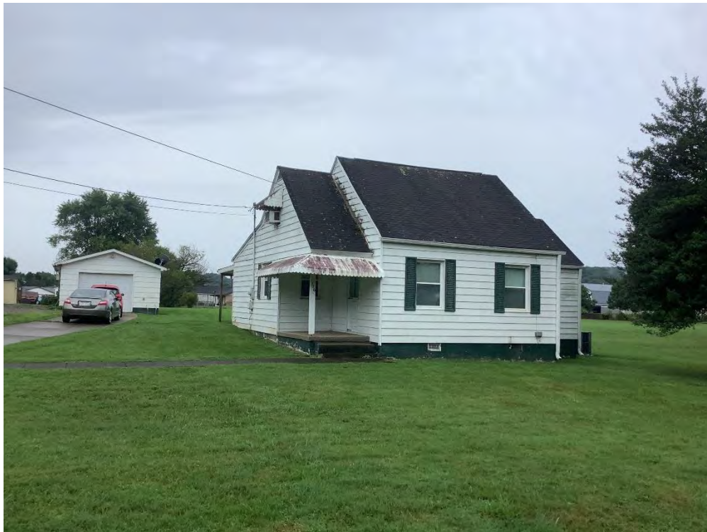
Photograph 22. PU-0003-0399 at 116 Kapok Street, facing South.
