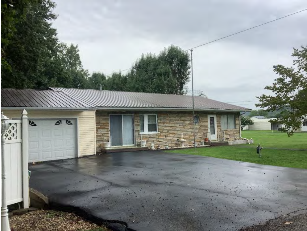
Photograph 27. PU-0007-0170 at 122 Kapok Street, facing South.
