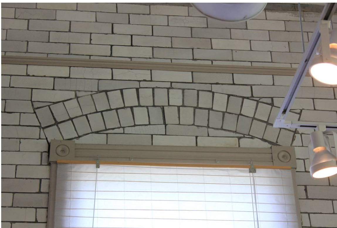
Photo #10: Interior: glazed tile brick and segmental arch lintel in main retail space, first floor
