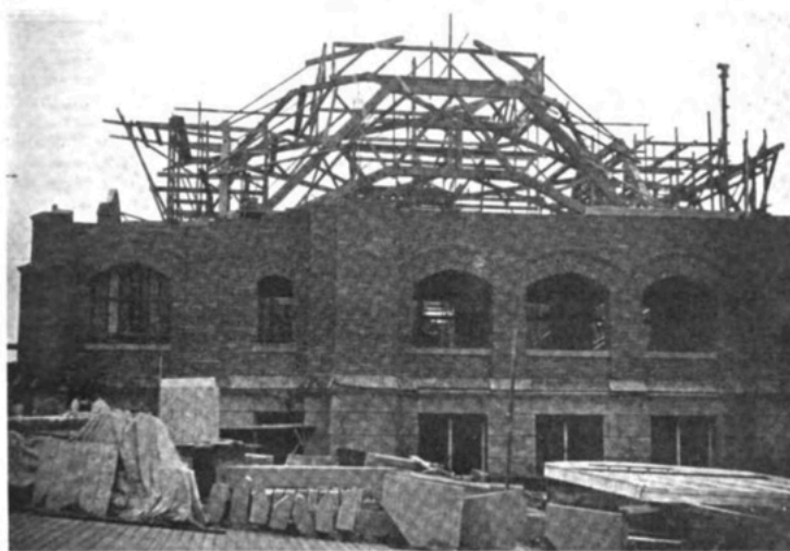
A VIEW OF SOME OF THE UNCOMPLETED FRAMING OF THE CHURCH DOME
