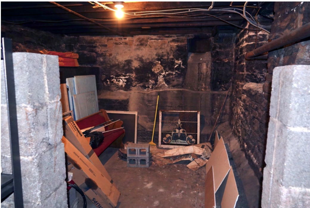
Photo 50. FUMC_050 – View of furnace room, located beneath the fellowship hall, facing southeast. A cinder block coal bunker, shown here, takes up the south corner of the room.
