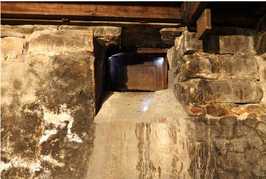
Photo 52. FUMC_052.tiff – Close-up of coal chute, facing southeast.
