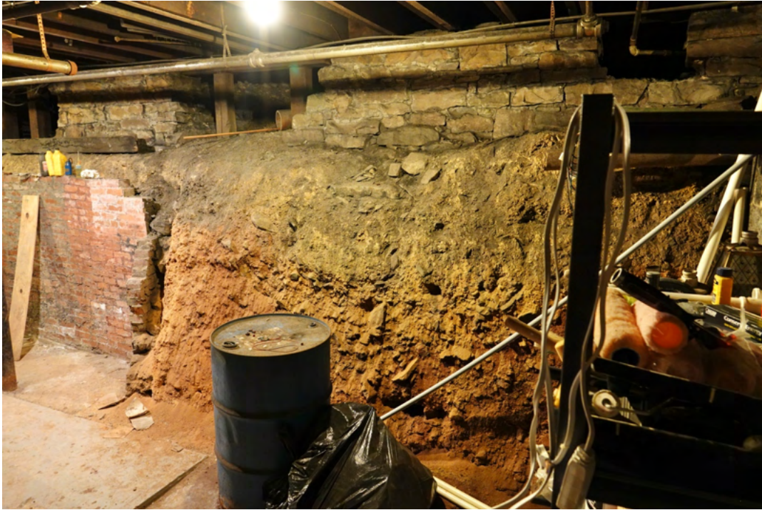
Photo 51. FUMC_051.tiff – View of furnace room, located beneath the fellowship hall, facing north. Floor joists, stone and earth foundations, and brick retaining wall visible.
