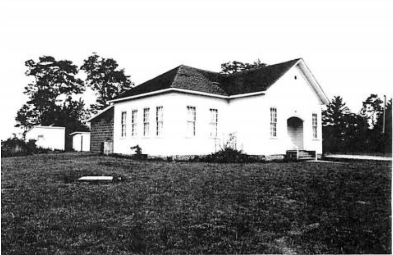
Figure 5. 1995 Photograph from WV SHPO Historic Property Inventory Form. Shows original 9/9 sash windows and the former asphalt shingle roof. From Wyoming/ Cloverdale Transmission Line Survey, #C9-5, ME-0294.
