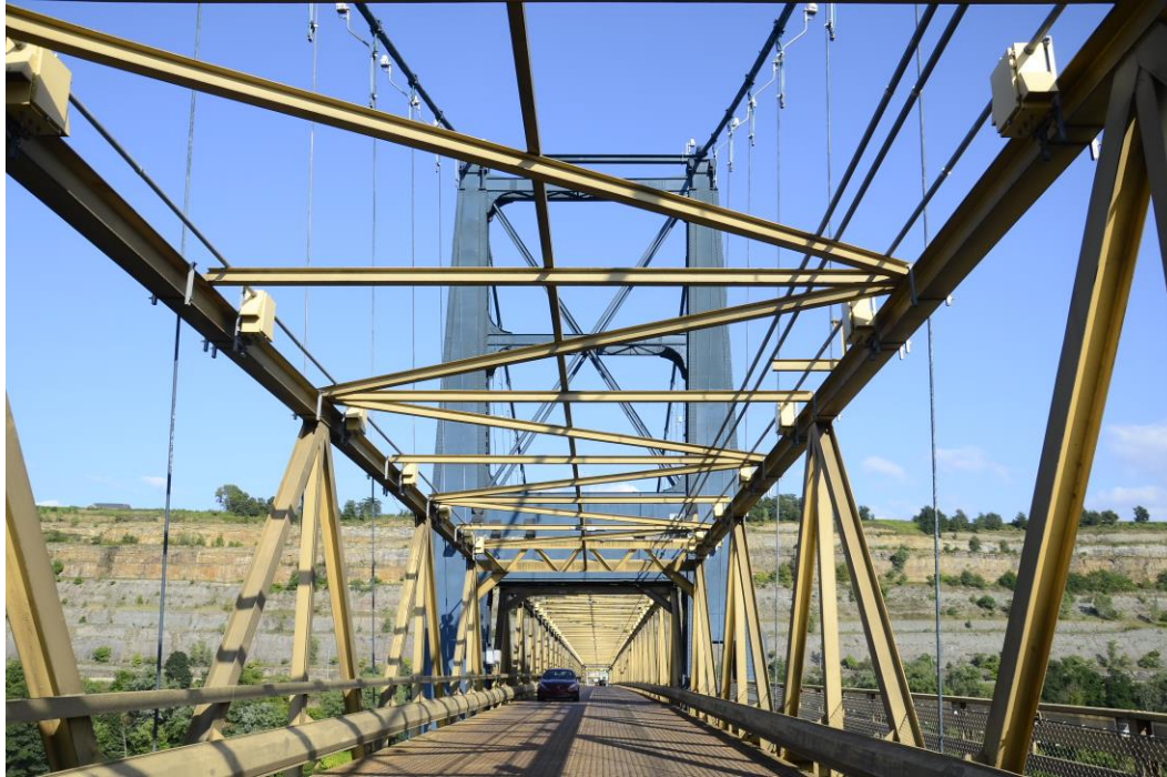
Photo 11: Market Street Bridge, Detail of the western side of the Ohio tower, facing east
