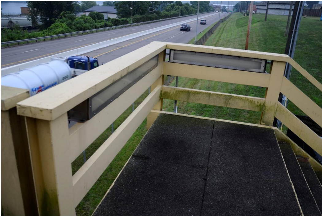
Photo 7: Market Street Bridge, Handrail & Stair landing, Note lighting under Handrail Cap, facing South
