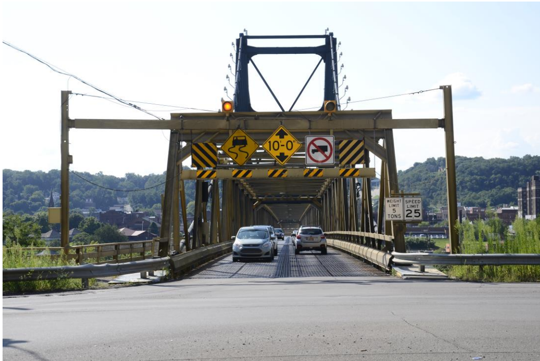
Photo 9: Market Street Bridge, approach on the WV (eastern) side of the river, facing west
