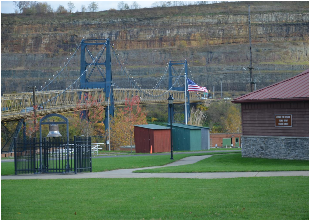
Photo 3: Market Street, Facing SE, taken while standing at Fort Steuben, Ohio
