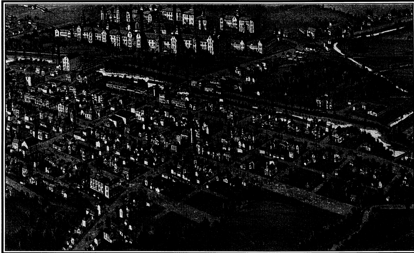
Fig. 1 This detail from the 1910 T. M. Fowler bird's eye view of the community shows the majority of the district as it existed at that time. Court Street was unopened beyond East Fourth Street and little existed north of Stone Coal Creek.
