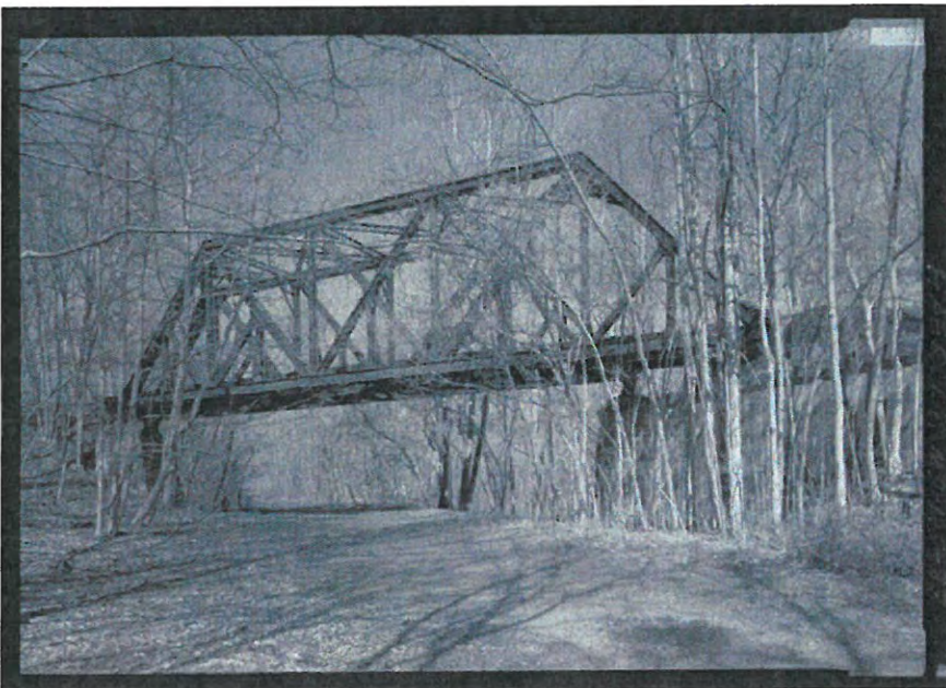
Photo 2 of 26 Railroad Bridge No. 1363, south elevation
