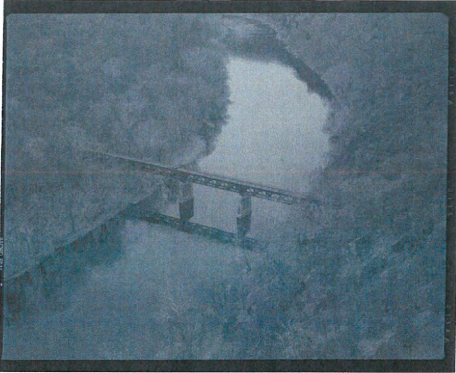
Photo 5 of 26 Railroad Bridge No. 1407, view west
