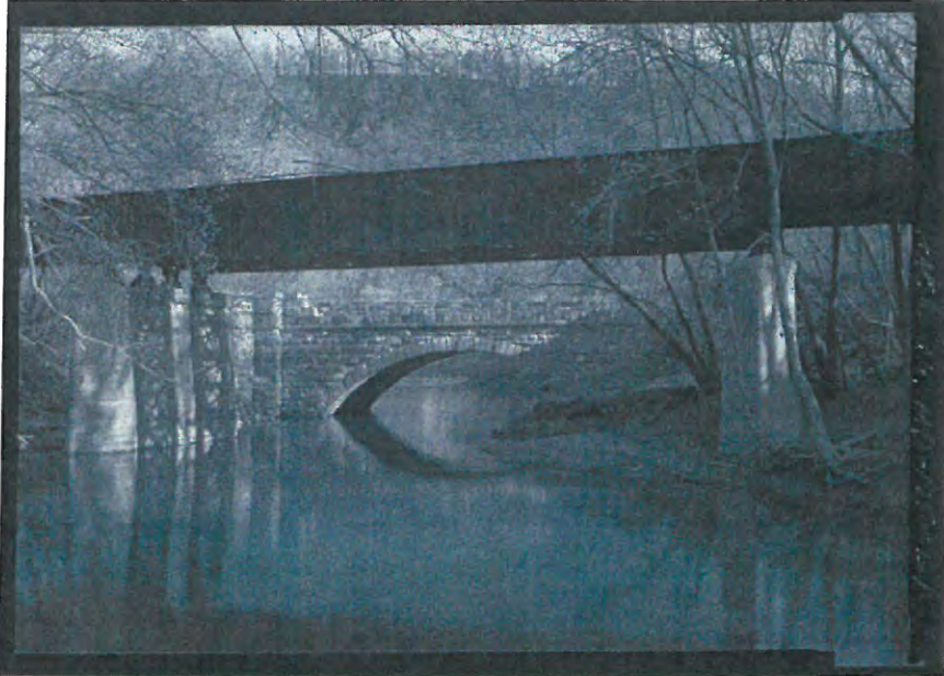
Photo 7 of 26 Railroad Bridge No. 1474, view south
