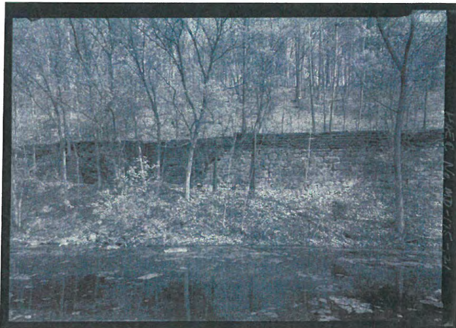
Photo 19 of 26 Railroad Retaining Wall 14, view north
