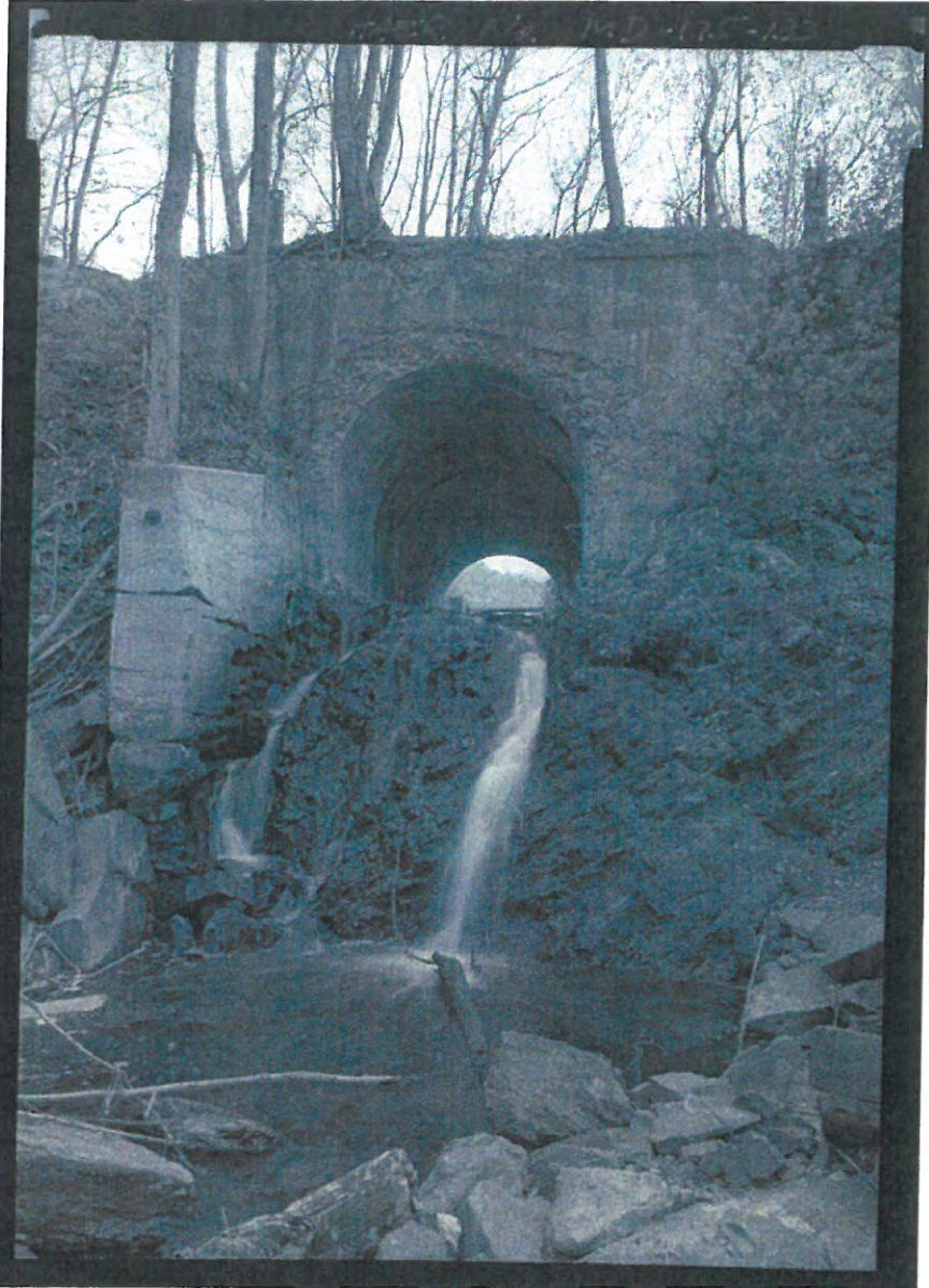
Photo 12 of 26 Railroad Culvert 144, view south
