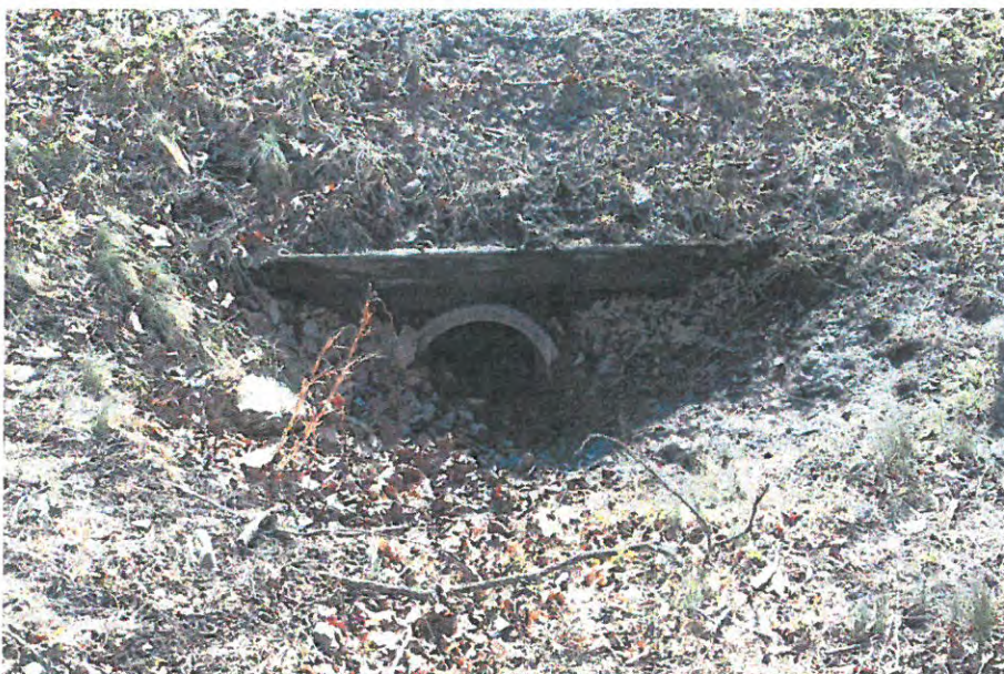
Photo 14 of 26 Railroad Culvert 166, north elevation
