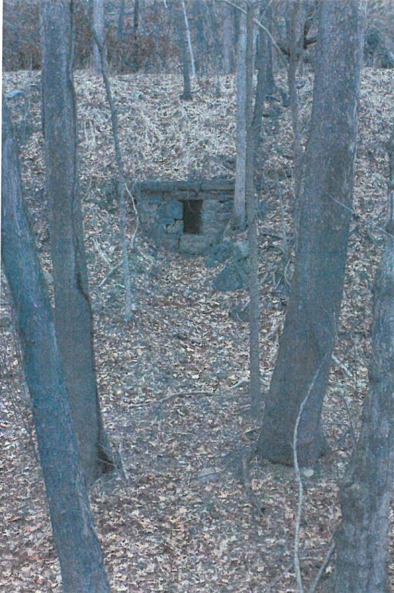
Photo 11 of 26 Railroad Culvert 94, view north
