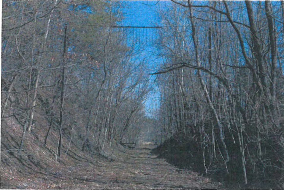
Photo 26 of 26 Railroad Tell-Tale, west elevation view
