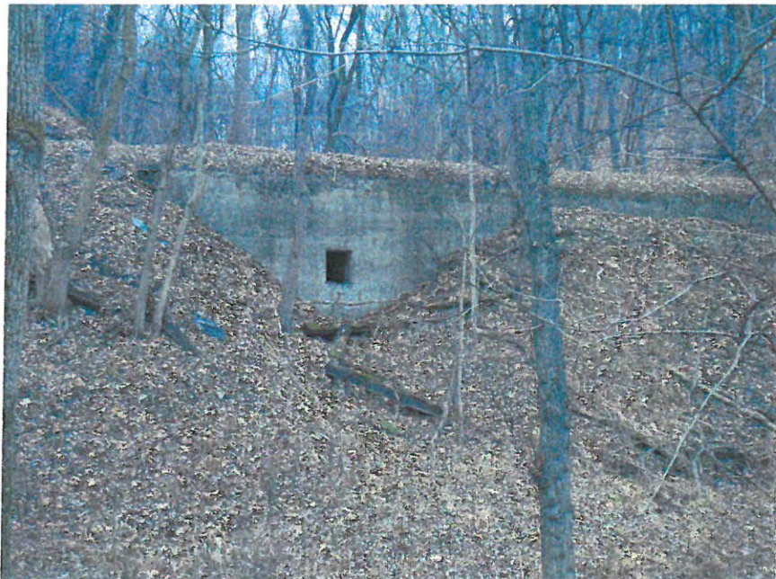
Photo 8 of 26 Railroad Culvert 12, view north
