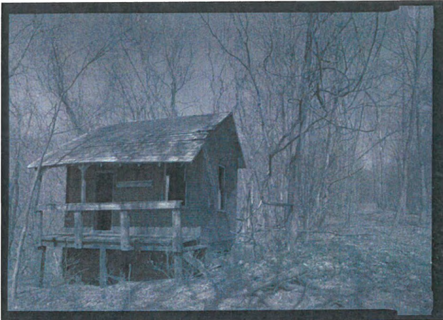
Photo 22 of 26 Jerome Telegraph Office, view north
