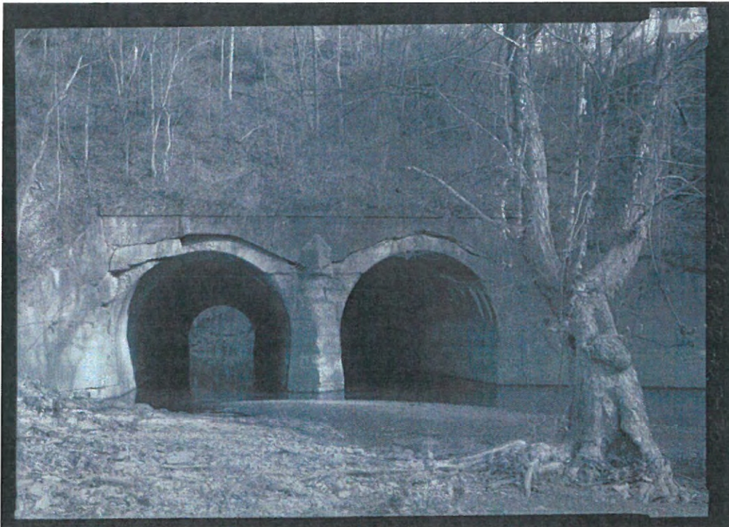
Photo 9 of 26 Railroad Culvert 22, view southeast
