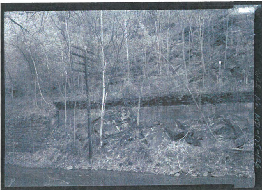
Photo 23 of 26 Railroad Retaining Wall 19, view north
