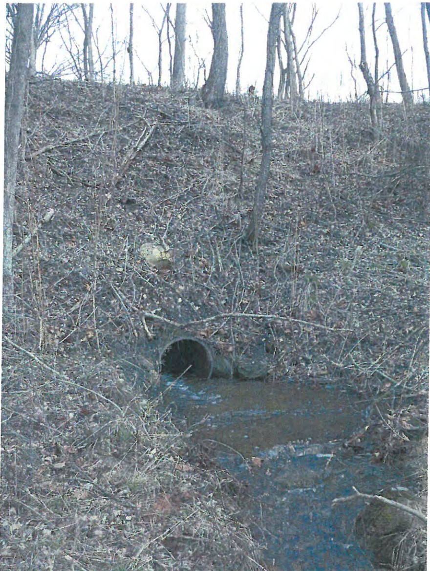
Photo 10 of 26 Railroad Culvert 73, view south
