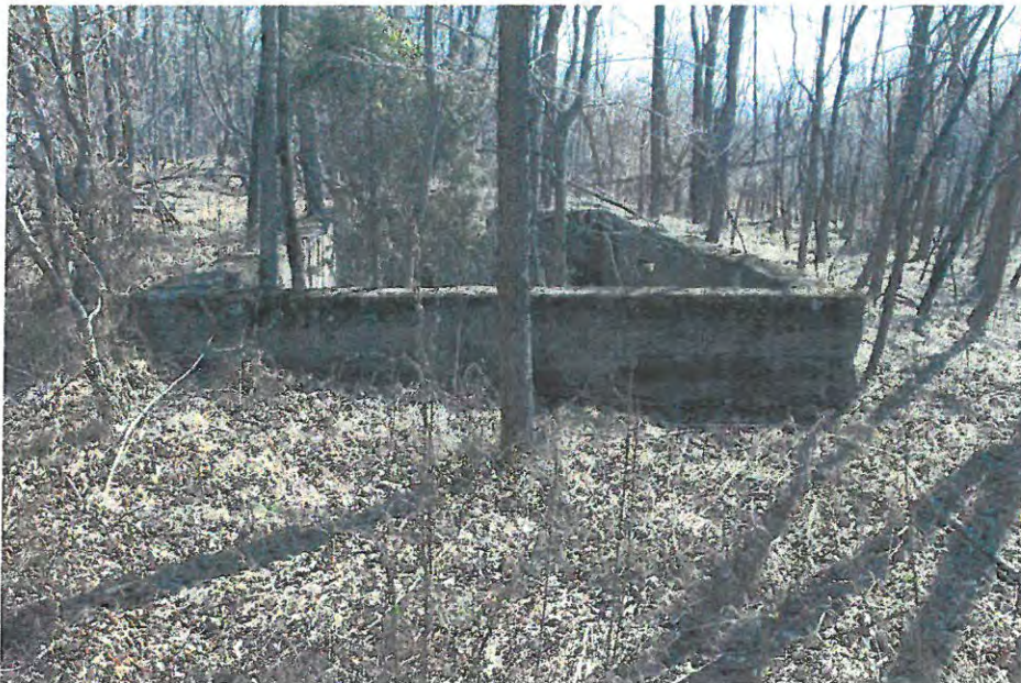
Photo 25 of 26 Railroad Section Foreman's Dwelling, Foundation, northeast elevation
