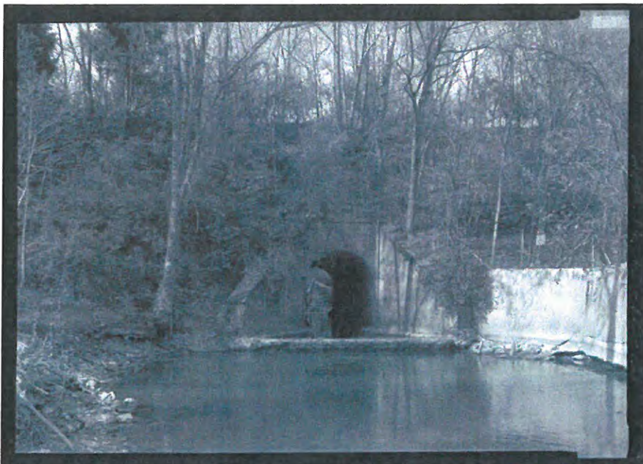
Photo 13 of 26 Railroad Culvert 128, view north
