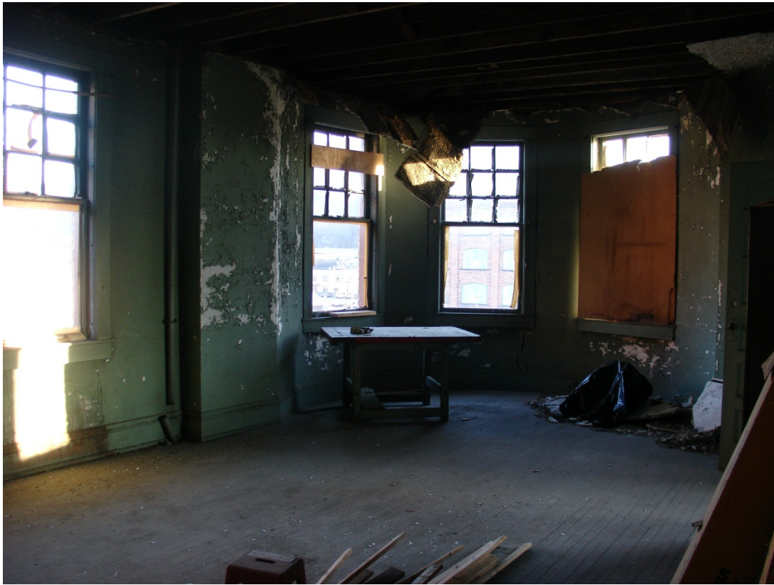
Photo 14: Fifth floor interior (c.1907 addition)
