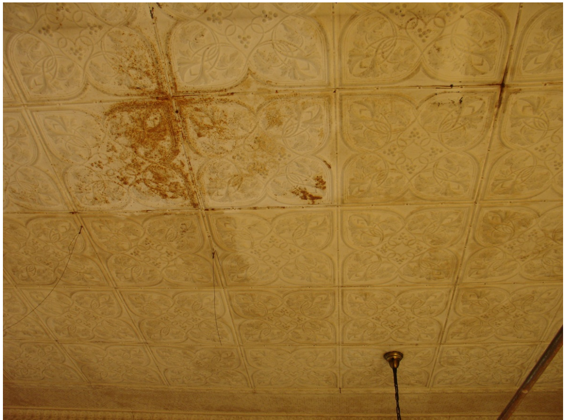
Photo 10: Third floor ceiling
