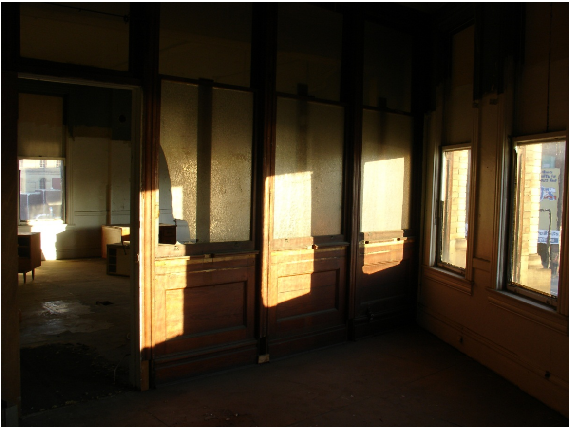
Photo 14: Fourth floor, interior room partition
