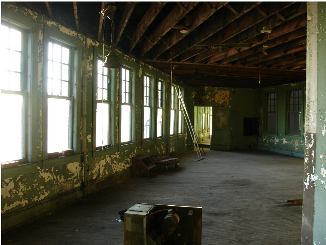
Photo 15: Fifth floor interior (c.1907 addition)
