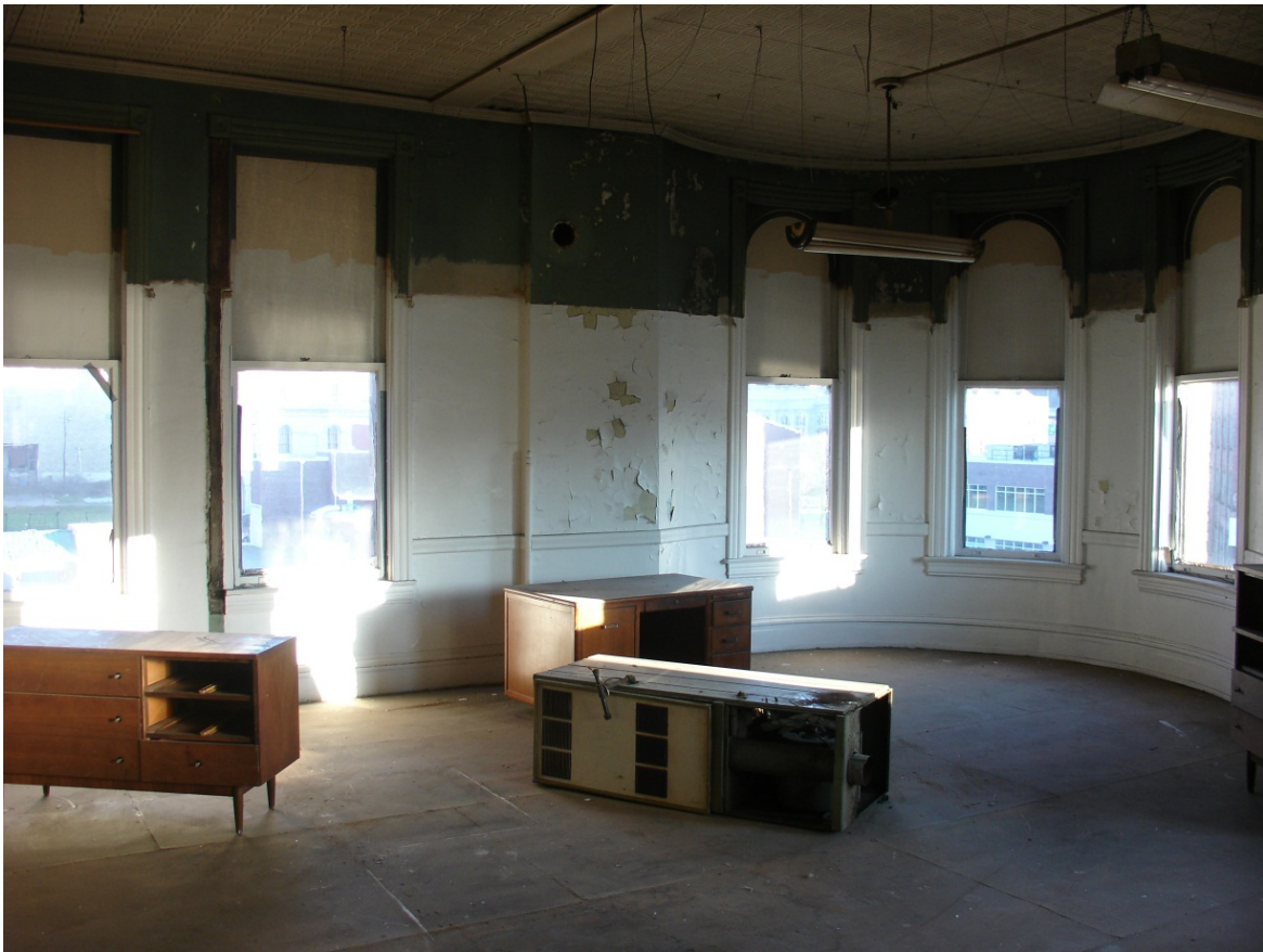
Photo 13: Fourth floor interior showing rounded building corner
