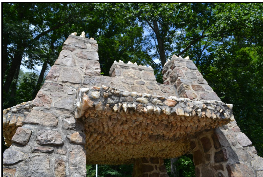
Figure 5: Detail, Top of Pin Oak Fountain, East Side, Showing crenellation and quartz detailing.
