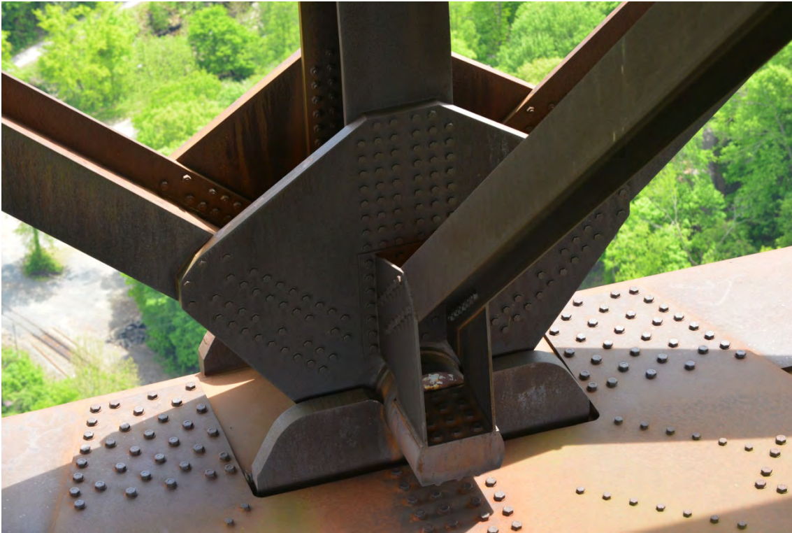
Photo 9 of 14 Center inverted A-frame member between center of arch and deck truss.
