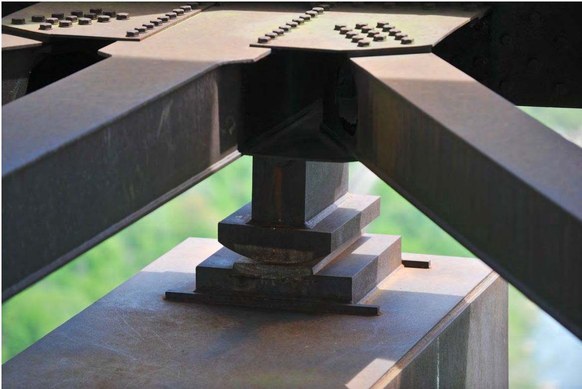
Photo 11 of 14 Example of a rocker shoe.
