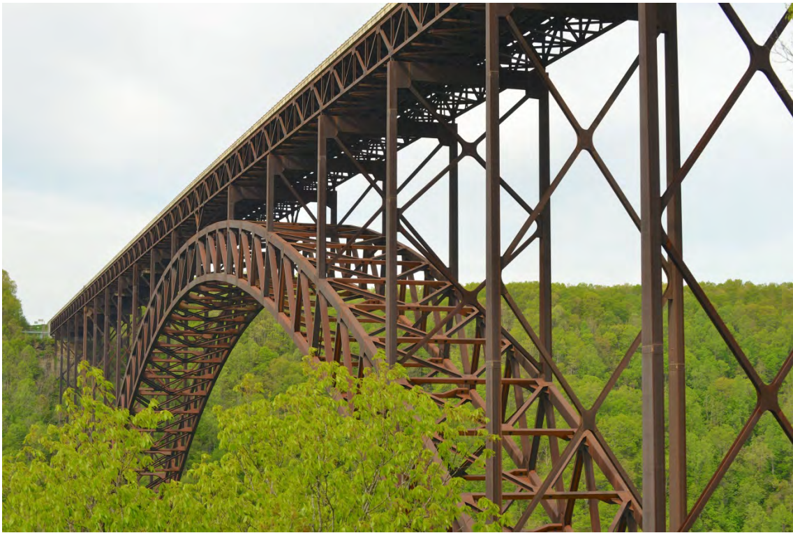
Photo 3 of 14 Arch, bents, and deck truss detail (see cross sections between column bents), facing west
