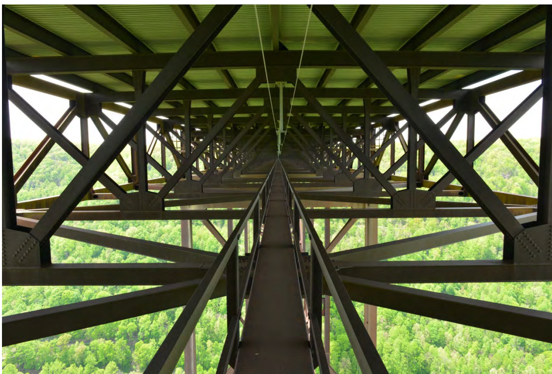
Photo 7 of 14 Inside deck truss showing catwalk, stringers, and floor beams, facing southwest.
