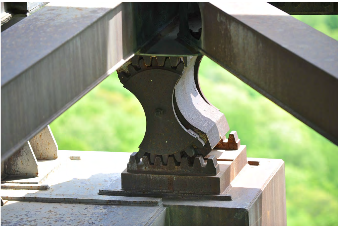
Photo 10 of 14 Example of expansion joint (gear configuration).
