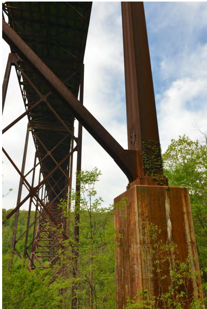
Photo 12 of 14 Bent 21, downstream column (showing cross bracing between bents), facing southwest.
