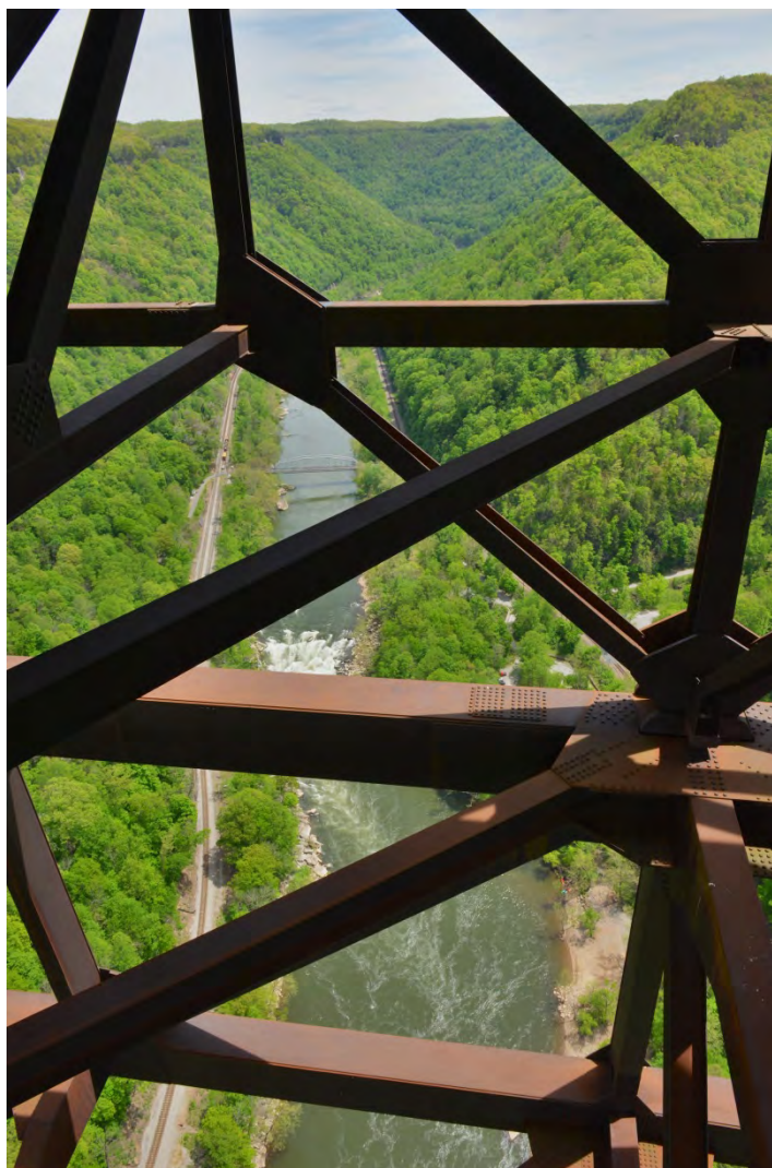
Photo 8 of 14 Truss members of deck truss and center inverted A-frame member, facing southeast.
