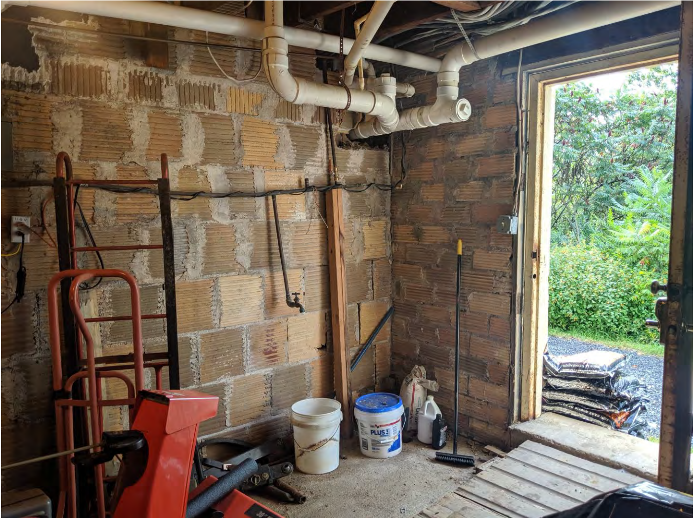
Photo 9. Interior view of 1915 terra cotta block foundation construction from basement, facing southeast.
