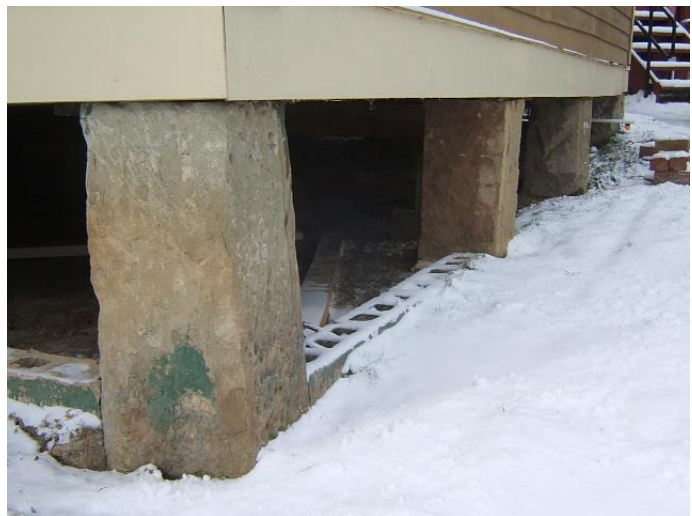
Photo 6: Foundation Pier Stones
