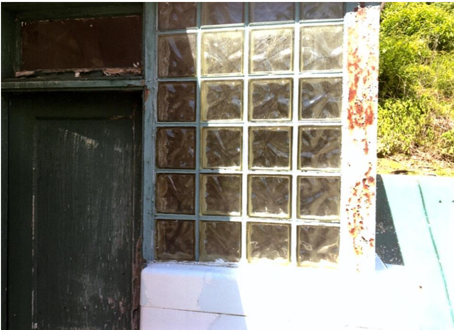
Photo 6: East Elevation, Glass block partition, facing north
