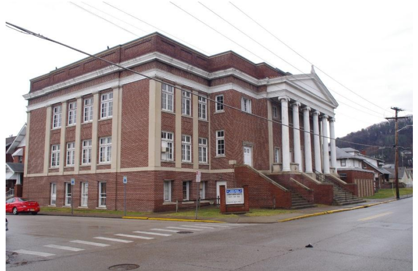
4. Resource #110. 501 Elizabeth Street looking northwest.
