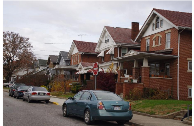
6. Resources #126-130. North side of Jackson Street looking northwest.
