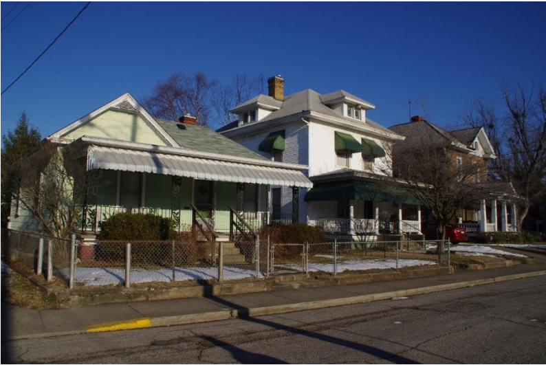
17. Resources #516-518. West side of Thompson Street looking west.
