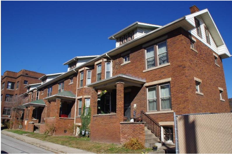
5. Resource #111. North side of Franklin Avenue looking northwest.
