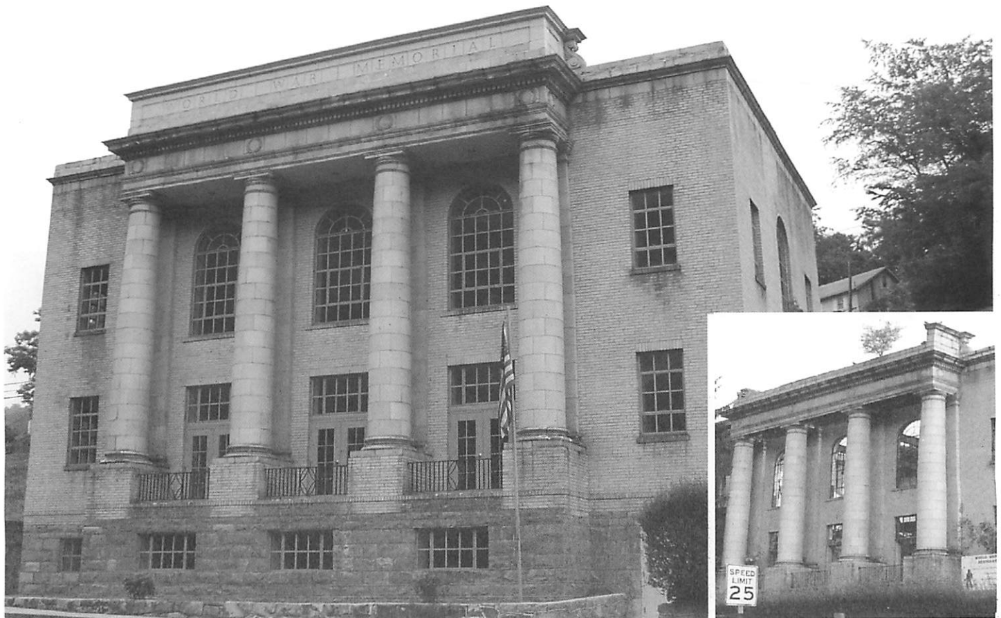
The restored Kimball War Memorial. Inset: Before renovations.
