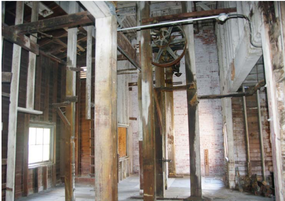
Photo# 14 - Penthouse Fl North Side Interior Facing East
