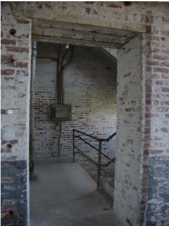
Photo# 08 - 2nd Fl Stairwell Landing Facing South
