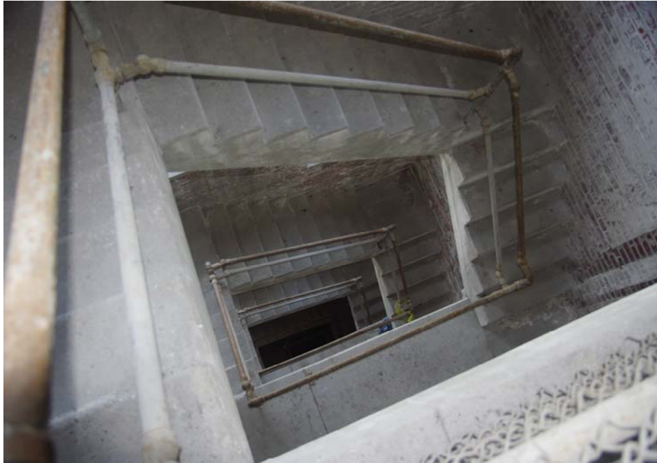
Photo# 13 - Stairwell Facing Down To Bottom Floors
