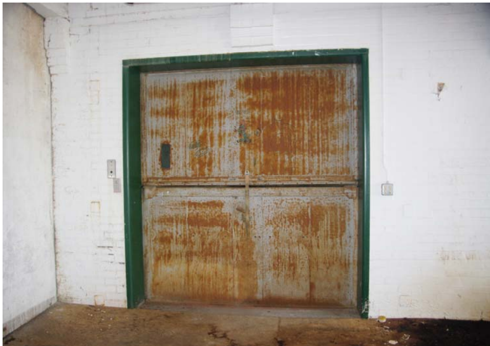
Photo# 12 - 5th Fl Southwest Room Elevator Door Facing South
