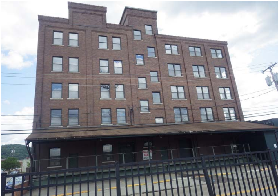
Photo# 01 - Front Façade Facing East
