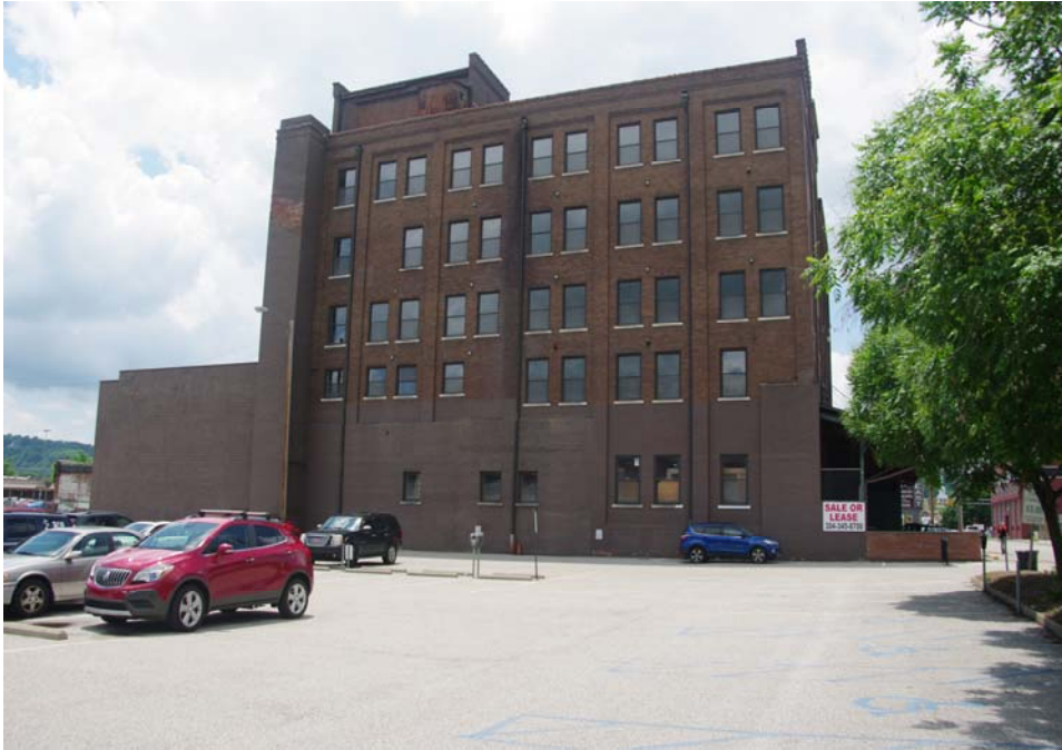
Photo# 05 - North Elevation Facing South
