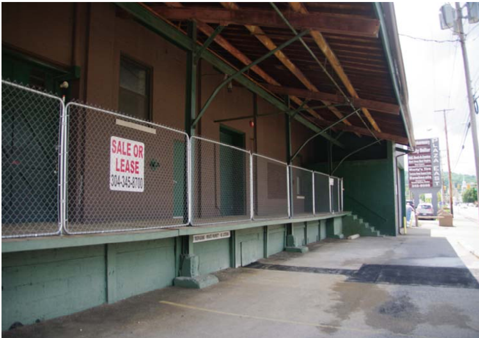
Photo# 16 - Front (west) Façade Loading Dock Facing South
