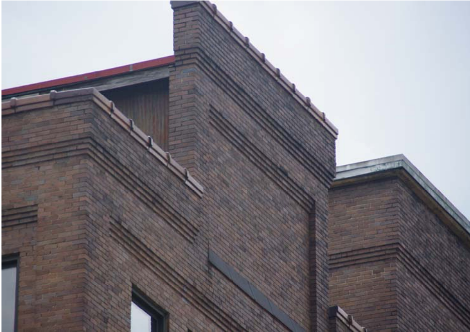
Photo# 07 - Detail of Cornice and Parapet at Northwest Corner of Building
