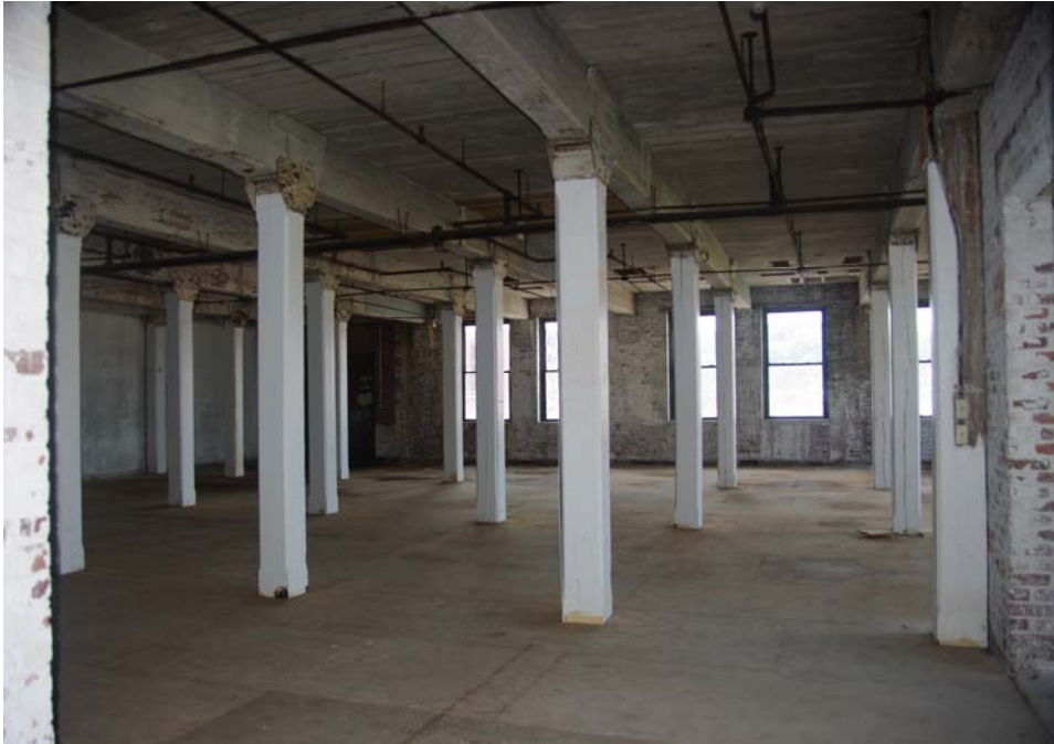
Photo# 09 - 3rd Fl Southwest Room Facing South
