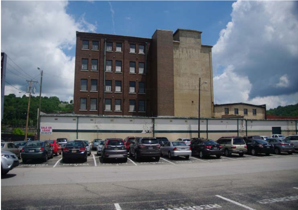
Photo# 03 - South Elevation Facing North
