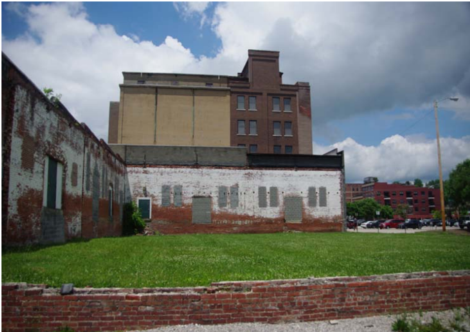
Photo# 04 - East Elevation Facing West
