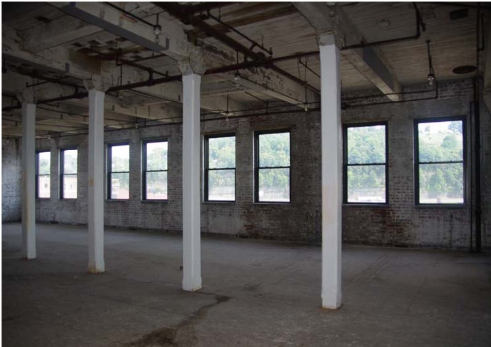
Photo# 10 - 5th Fl Northwest Room Facing Northwest
