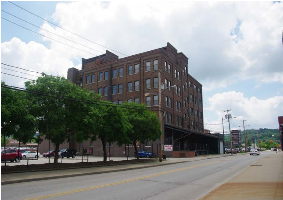
Photo# 06 - North Elevation Facing Southeast
